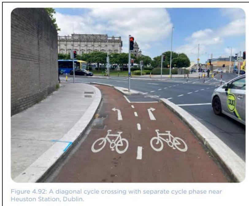
Figure 4.92: A diagonal cycle crossing with separate cycle phase near Heuston Station, Dublin.
