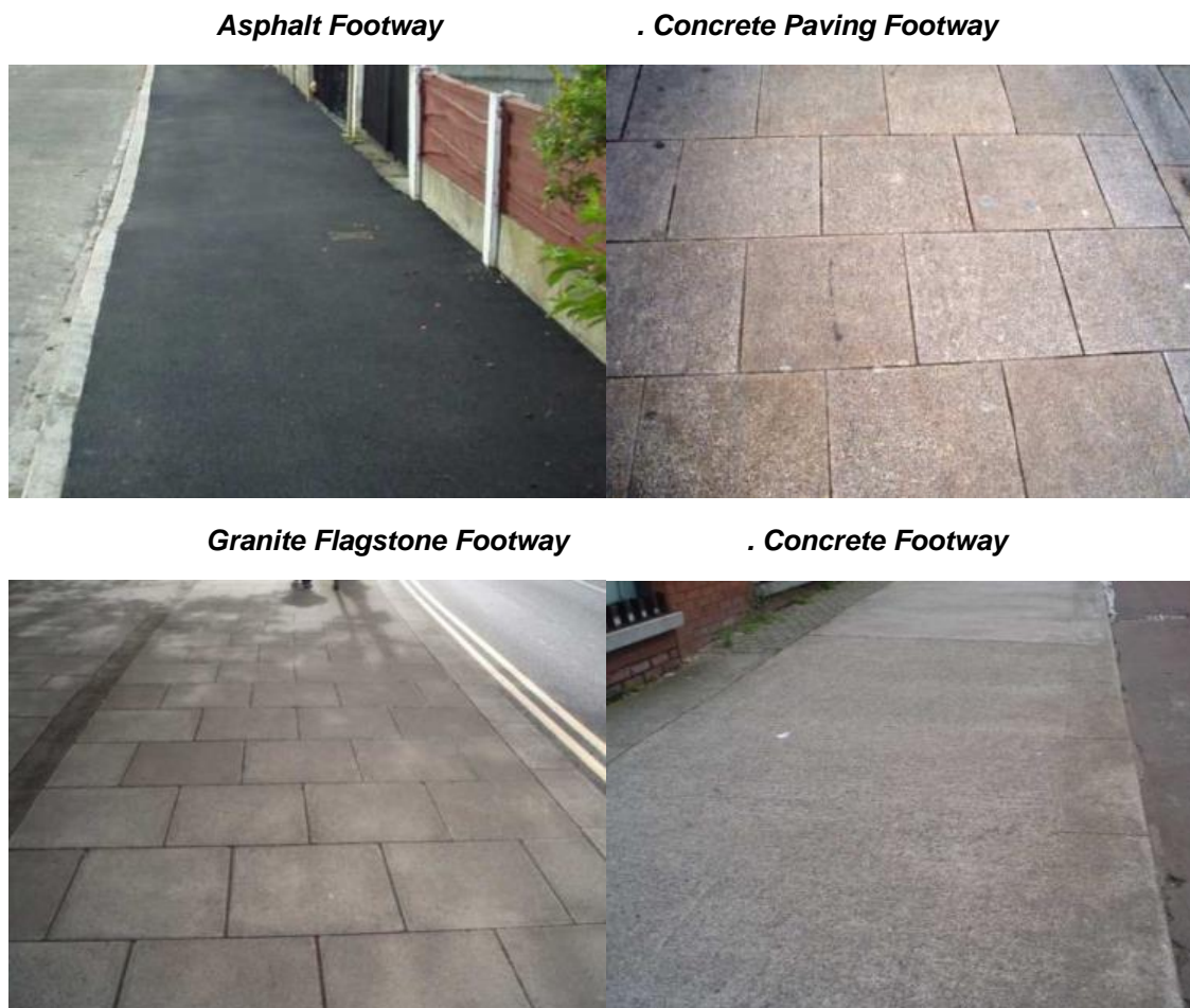
Figure 7-10: Footway Paving Types
