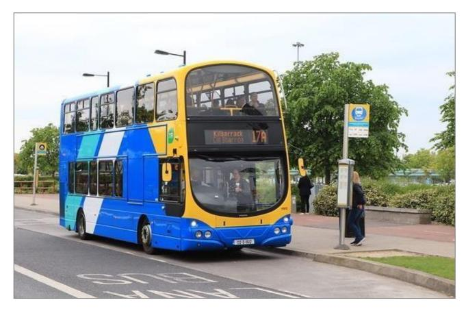
**Figure 1.6** A typical bus lay-by adjacent to a bus lane; note concrete surface for additional durability.
