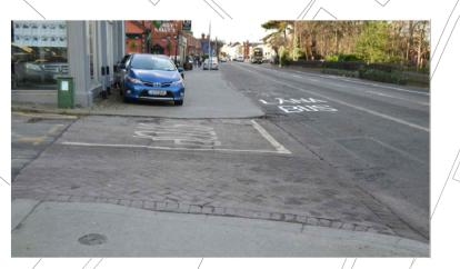
UNCONTROLLED/CROSSING POINT/WITH NO KERB DISPOSED IN JUNCTION WITH A SIDE ROAD. A/DISHED KERB AND BUFF" OR GREY TACTILE PAVING SHOULD BE CONSIDERED (FOR AN IN LINE CROSSING). DEPTH OF 1.2 M, GRADIENT 1:12 MAX. LEVEL DIFFERENCE OF DISHED KERB: 6MM. THE CRACKED PAVING IN THE CARRIAGEWAY OF THE SIDE ROAD SHOULD BE REPAIRED.
