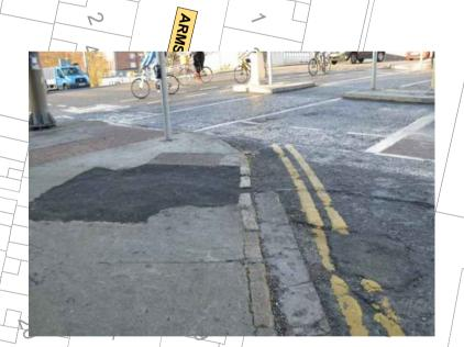
PATCHED FOOTPATH WITH ASPHALT IN THE UNCONTROLLED CROSSING POINT. PAVING SURFACE SHOULD BE REPAIRED AND TACTILE PAVING TO BE PROVIDED IN THE CROSSPOINT
