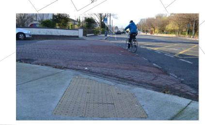
UNCONTROLLED CROSSING POINT AT SIDE ROAD. HIGH UPSTAND IN THE INTERSECTION WITH THE CARRIAGEWAY. LEVEL DIFFERENCE BETWEEN SURFACES SHOULD BE LESS THAN 6MM.
