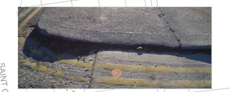
UNCONTROLLED CROSSING WITH A HIGH UPSTAND. LEVEL DIFFERENCE SHOULD BE HIGHER THAN 6MM IN THE DISHED KERB WITH THE CARRIAGEWAY. ABSENCE OF TACTILE PAVING
