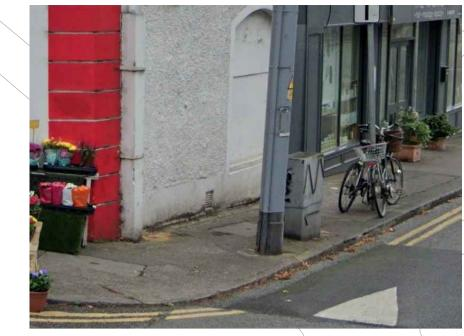
REDUCED WIDTH OF THE FOOTPATH DUE TO THE POSITION OF THE LIGHTING COLUMN AND THE ELECTRICITY BOX. A MINIMUM DISTANCE OF 1200MM IN A LENGHT OF 2000MM. SHOULD BE ENSURED.
