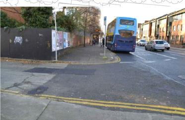
UNCONTROLLED CROSSING POINT WITH NO KERB DISPOSED. A DISHED KERB AND BUFF, OR GREY TACTILE PAVING SHOULD BE CONSIDERED (FOR AN IN LINE CROSSING). DEPTH OF 1.2 M, GRADIENT 1:12 MAX. LEVEL DIFFERENCE OF DISHED KERB: 6MM. THE CRACKED PAVING IN THE CARRIAGEWAY OF THE SIDE ROAD SHOULD BE REPAIRED
