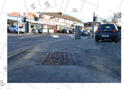
DETERIORATING PAVING AROUND A IRON GRID COVER IN THE DIRECT LINE OF THE FOOTPATH. PAVEMENT CRACKED SHOULD BE REPAIRED TO BE FIRM AND HARD-
