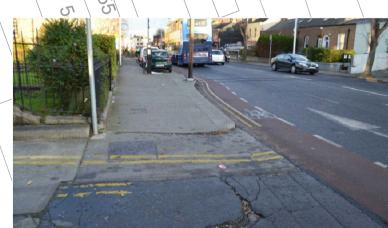
UNCONTROLLED CROSSING POINT WITH NO KERB DISPOSED. A DISHED KERB AND BUFF" OR GREY TACTILE PAVING SHOULD BE CONSIDERED (FOR AN IN LINE CROSSING). DEPTH OF 1.2 M, GRADIENT 1:12 MAX. YLEVEL DIFFERENCE OF DISHED KERB: 6MM. THE CRACKED PAVING IN THE CARRIAGEWAY OF THE SIDE ROAD SHOULD BE REPAIRED.
