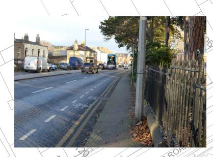
REDUCED WIDTH IN THE FOOTPATH ADJACENT TO HAROLD CROSS PARK. A MINIMUM WIDTH OF THE POOTPATH OF 1500MM. SHOULD BE ENSURED AND 1200MM. IN SOME POINTS IN A LENGTH OF 2000MM
