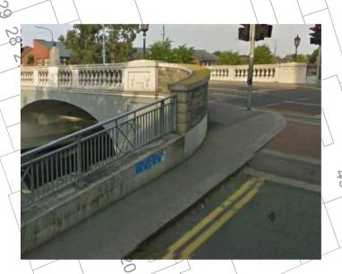
GRADIENT AND WIDTH OF THE FOOTPATH SHOULD BE CHECKED. IF GRADIENT IS <1:20 (5%) IT SHOULD BE CONSIDERED AS A RAMPED ROUTE AND ACCESSIBILITY MEASURE TO BE PROVIDED A 1500 MM. MINIMUM WIDTH OF FOOTPATH WHEN OBSTACLES CAN NOT BE REMOVED AND HANDRAILS SHOULD BE PROVIDED IF NECESSARY.
