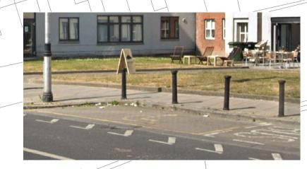
ON-STREET ACCESSIBLE CAR PARKING BAY A DROPPED KERB SHOULD BE INCORPORATED FOR ACCESSING TO THE FOOTPATH. IN THE DESIGN PROJECT, A CYCLE TRACK IS PROPOSED IN THIS AREA PARALLEL TO THE BUS STOP. A SUITABLE SPOT FOR THIS PARKING BAY SHOULD BE LOCATED, IF THIS IS REMOVED FOR THE NEW STATE OF CARRIAGEWAY. CHECK DIMENSIONS. 7M LONG AND PREFERABLY 3.6M WIDE. FOR A DESIGNATED ON-SITE PARALLEL PARKING BAY.
