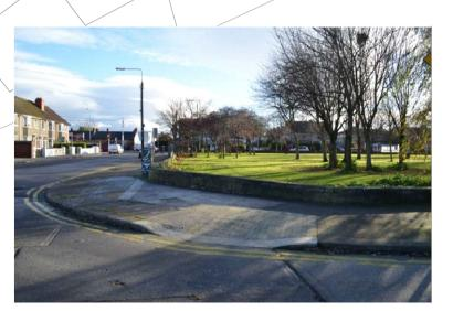
UNCONTROLLED CROSSING POINT WITH NO DISHED KERB AND TACTILE PAVING PROVIDED. A DISHED KERB AND BUFF" OR GREY TACTILE PAVING SHOULD BE CONSIDERED (FOR AN IN LINE CROSSING). DEPTH OF 1.2 M, GRADIENT 1:12 MAX. LEVEL DIFFERENCE OF DISHED KERB: 6MM
