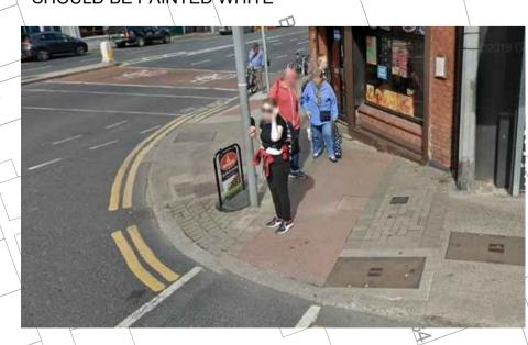
UNCONTROLLED CROSSING POINT AT A SIDE ROAD. CRACKED PAVING IN THE CARRIAGEWAY FOR CROSSING. THE PAVEMENT SHOULD BE REPAIRED AT THIS POINT WITH MINIMAL VERTICAL DEVIATIONS.
