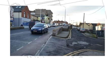
CHANGE IN LEVEL IN FOOTPATH. STUR ACCESSIBLE MEASURES FOR TERNAL STAIR. TACTIZE PAVING FOR THE UNCONTROLLED CROSSING SHOULD BE PROVIDED AND CORPUROY WARNING PAVING ALSO SHOULD BE DISPOSED IN THE START/ END OF THE STEPPED ROUTE 400 MM. AND HANDRAILS INCORPORATED.
