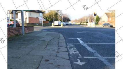
CONTROLLED CROSSING POINT WITH NO TACTILE PAVING AND PROPER KERB
